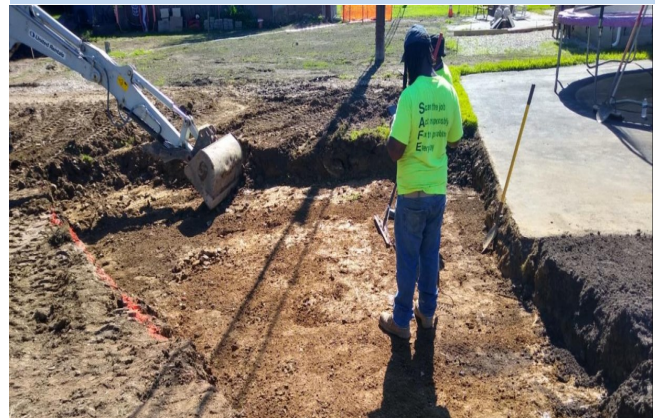
Above: Soil excavation at one of the affected properties August 2020
